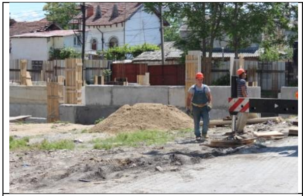
Construction continues on the UDG training facility for outreach to Muslims.
